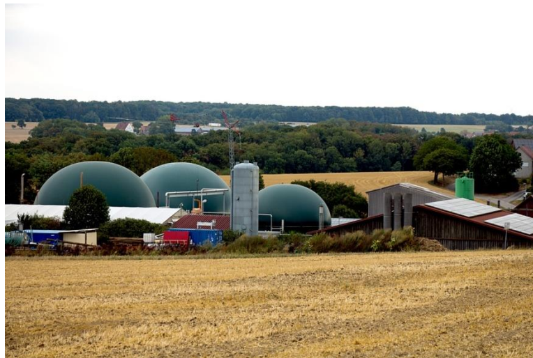
Figure 22: Biogas Plant Karle / Agro Energie Hohenlohe GmbH & Co. KG; blue containers in from: pilot plant for nutrient recovery (picture credit: IBBK Fachgruppe Biogas GmbH)
